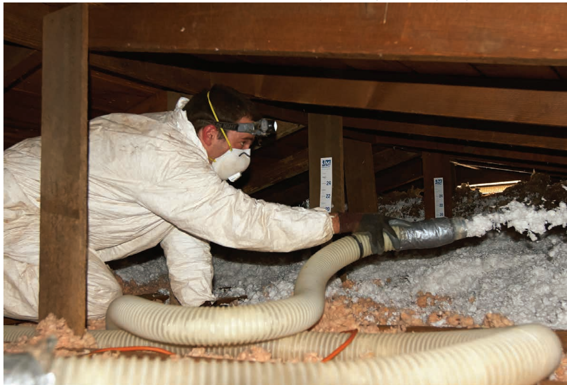
AIR SEALING AND INSULATION: The first step to improving an older home is air sealing and adding insulation to attic spaces.
