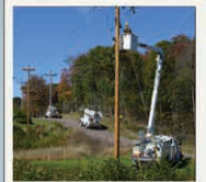
NEW CONSTRUCTION ALONG WEST MUD PIKE
