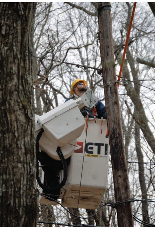
DE-ENERGIZING: Somerset REC Lineman Alex Mazanowski uses a "hot stick" to de-energize the line so other crew members can start their work safely on the next pole.
